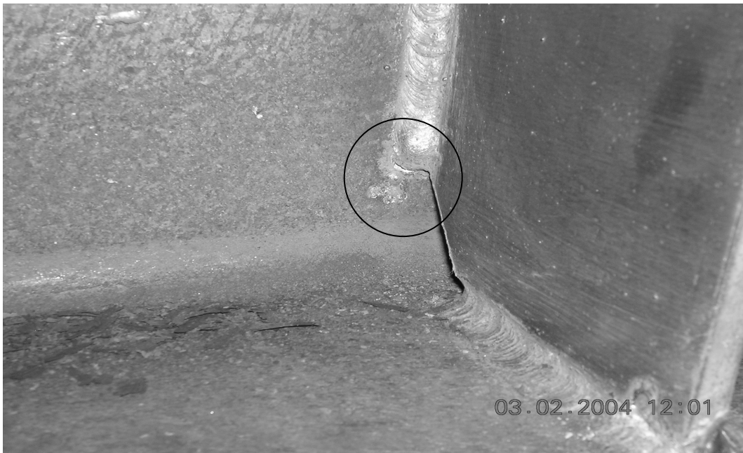
Figure 3.66 Specimen 10: Crack observed at the bottom of the north stiffener after the first cycle of load step 11 ( \gamma = +0.09 radian)
