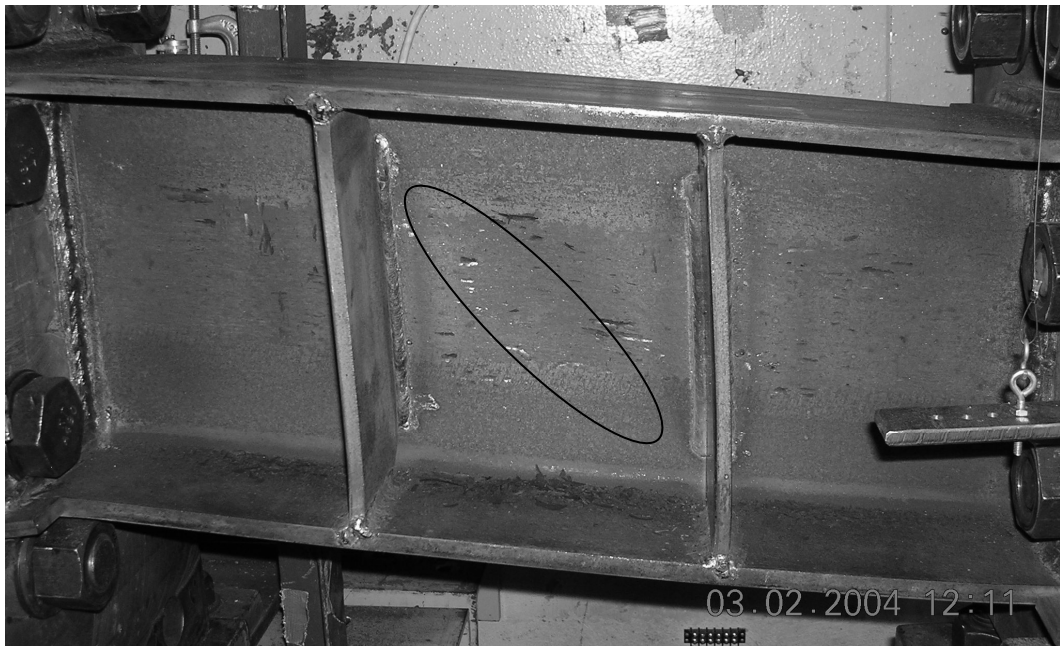
Figure 3.67 Specimen 10: Web buckling observed after the first cycle of load step 11 ( \gamma = -0.09 radian)
