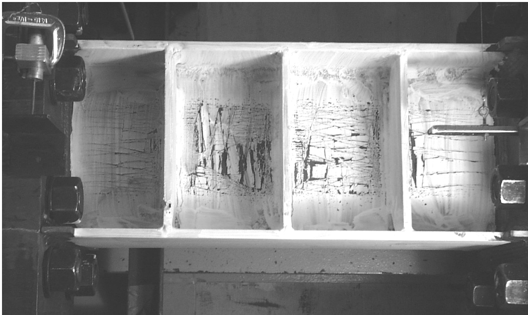
Figure 3.26 Specimen 2: Web yielding after the first cycle of load step 3 ( \gamma = +0.01 radian)
