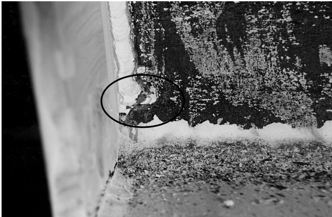
Figure 3.22 Specimen 1: Crack observed at the toe of the welding of the far north stiffener during the fourth cycle of load step 8 ( \gamma = -0.06 radian)
