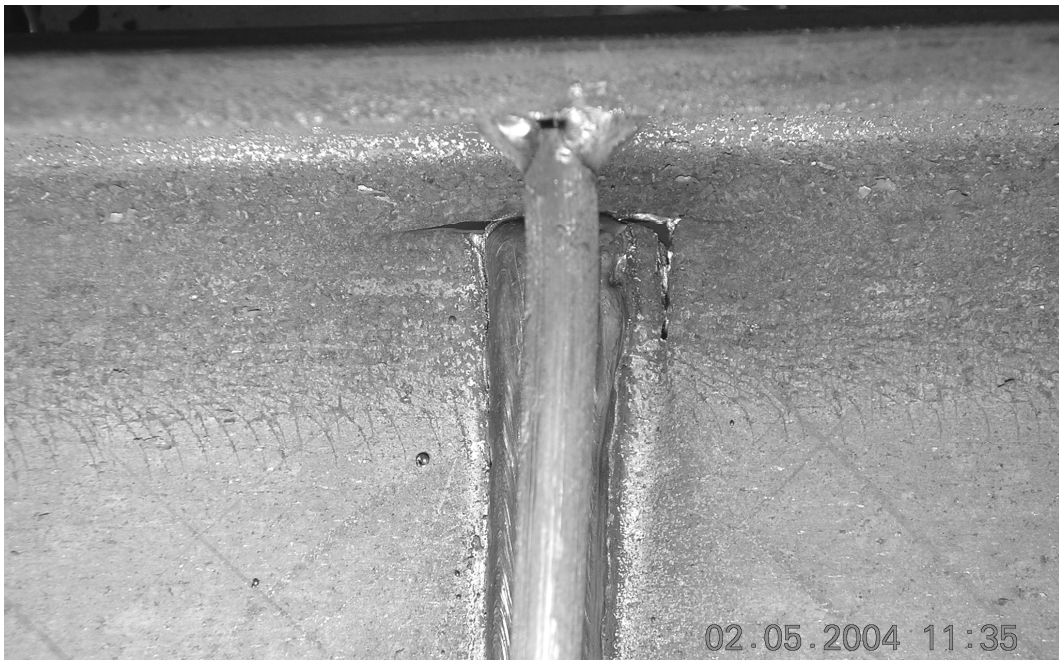
Figure 3.44 Specimen 6: Crack at the top of the center stiffener during the first Half of the third cycle of load step 8 ( \gamma = -0.06 radian)
