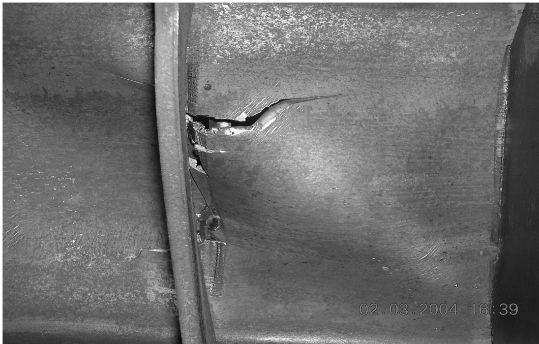
Figure 3.41 Specimen 5: Closer look at the crack formed behind the center stiffener after testing
