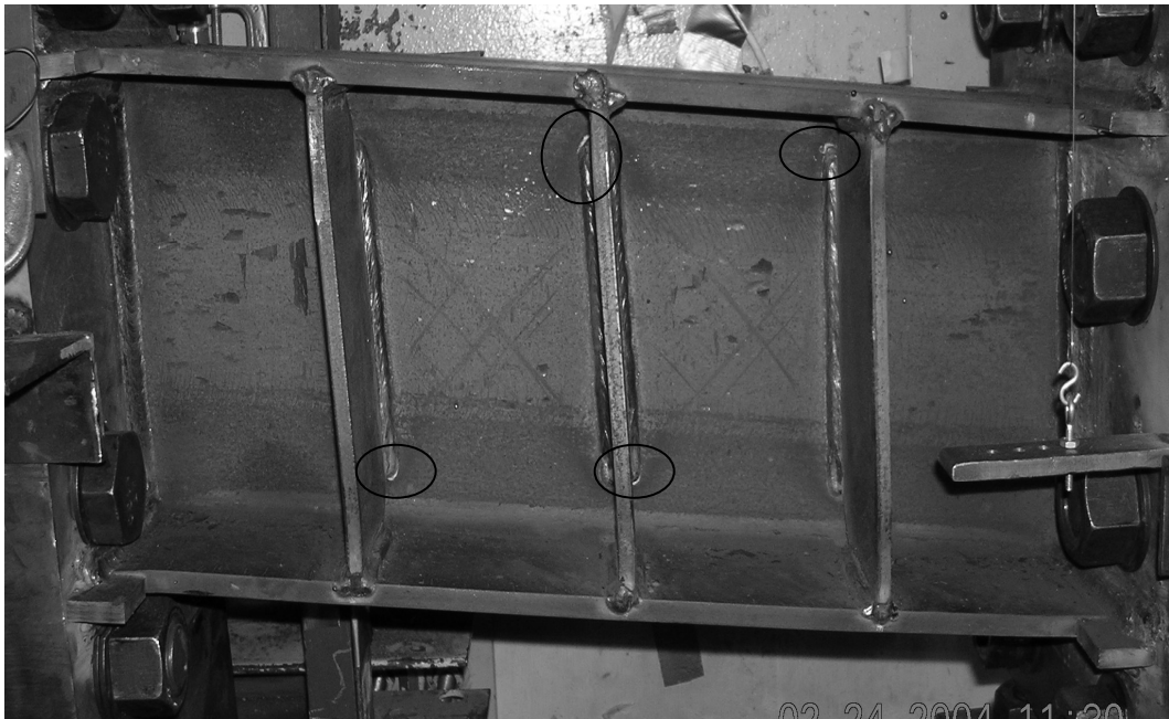
Figure 3.60 Specimen 9: Cracks observed after the first cycle of load step 11 ( \gamma = -0.09 radian)
